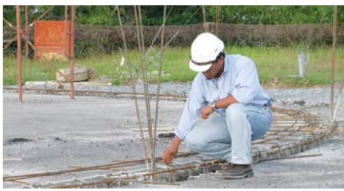
The ongoing civil ground works
